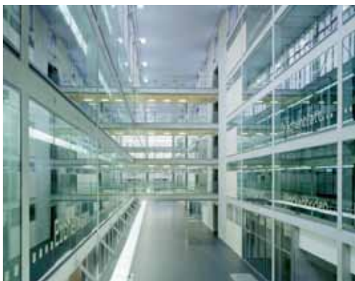
ZKB Steinfels, Zurich, CH, 18,000 m2 offices and 16 apartments. 2004 Photo: Andrea Helbling
