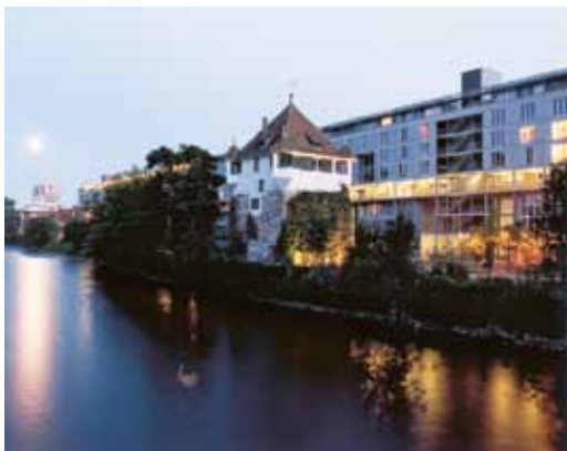
Limmatwest, Zurich, CH, 314 Apartments, Offices, Commercial, Retail. 2002 Photo: Gabriel Neukom
