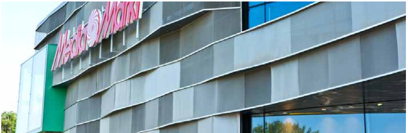
Silvery lace curtain to the main façade
